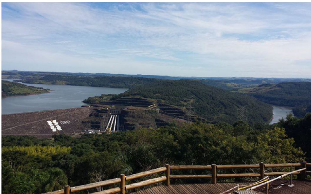
Figure 2 – View of the Segredo Hydroelectric dam, Facebook, source Guisla Schmickler.
