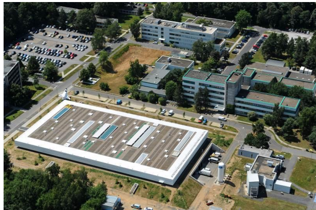
Figure 1: Location of :envihab in front of the DLR Institute of Aerospace Medicine (top right of :envihab) on DLR premises in Cologne, Germany, with six atria (blue stripes on the roof) to allow for the influx of daylight
