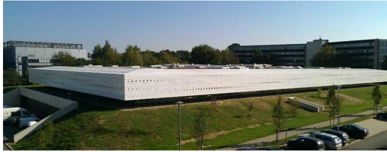
Figure 3: The massive white roof houses the technical infrastructure of :envihab. The main floor with its modules is a slightly bit dug into the ground
